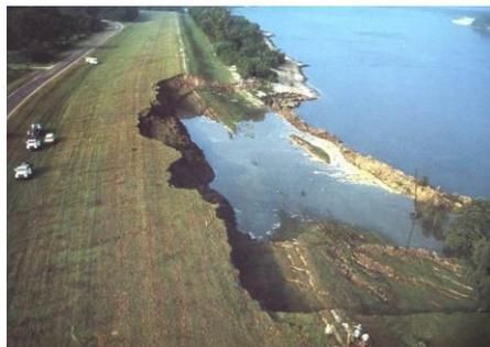
Figure 1 Example of damage to a river dike due to a flow slide (Rogers, 2012)
